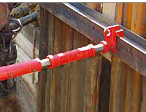
► End hooks for steel walings - special solution
